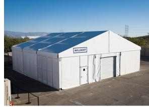
From simple industrial storage to beautiful event spaces, Pre-Engineered Clearspan structures are designed to meet needs across a wide range of projects. These rapidly deployable buildings are made from industrial fabric with engineered aluminum framing and can be installed nearly anywhere, on any surface.
